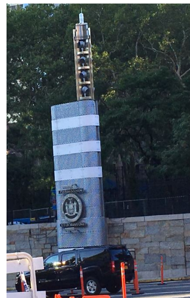
New decorative Tower at MTA Queens Midtown Tunnel, Manhattan side.
