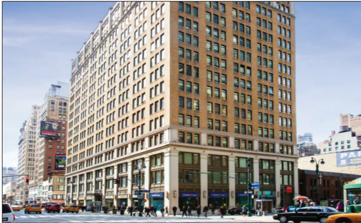
Figure G (Penn Terminal Building)
