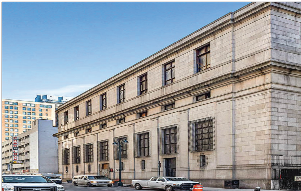
Figure H (Penn Station Service Building)
